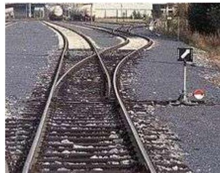
positions to direct a train coming from the point blades toward the straight path or the diverging path. A train moving from the narrow end toward the point blades is said to be executing a *facing-point movement*.
